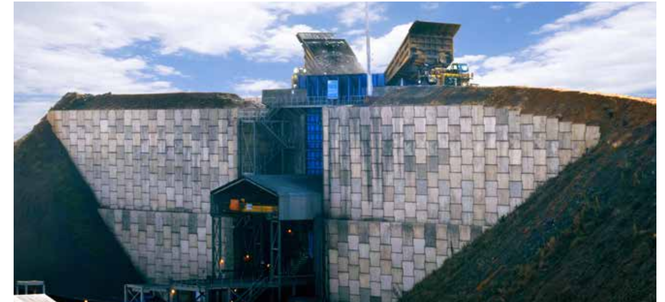
MacRes® concrete faced reinforced soil structure
