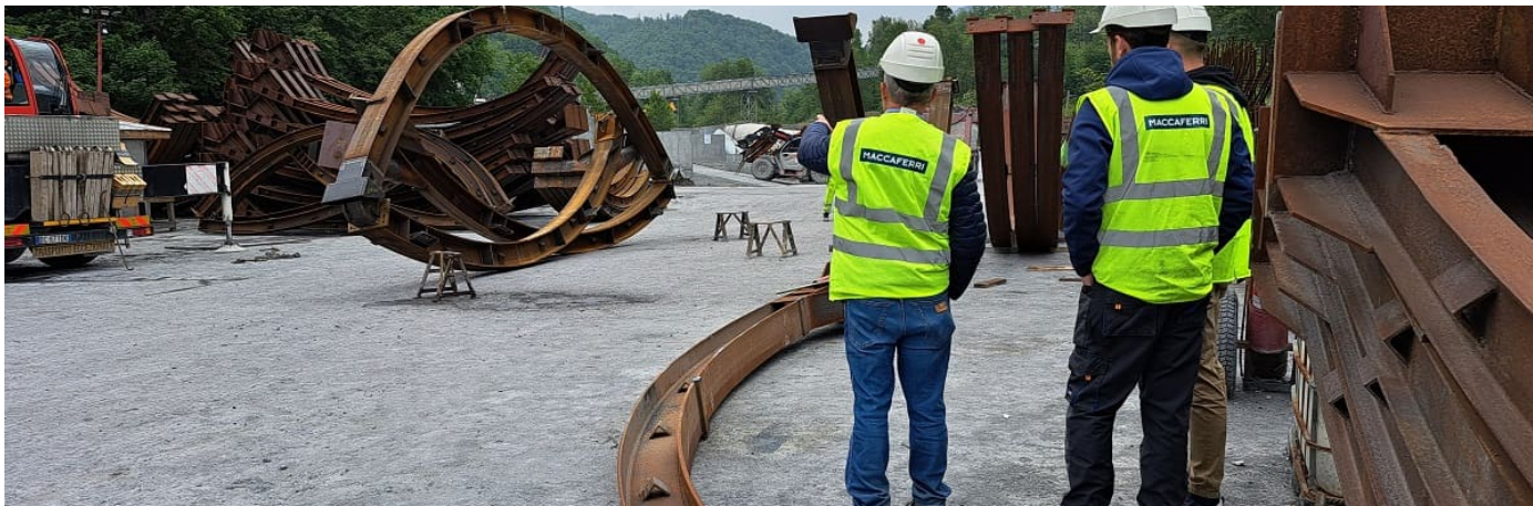
Pre-assembled Automated Tunnel Rib HEB300
