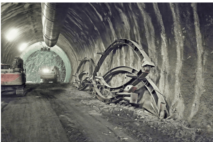
Pre-assembled Automated Tunnel Rib HEB300 before
