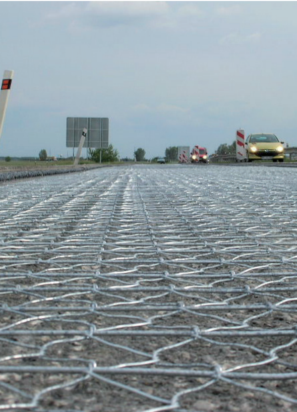
Road Mesh® provides lateral restraint to the asphalt which improves resistance to rutting and shoving
