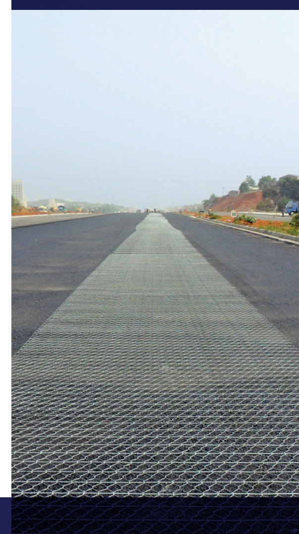
Road Mesh® - Structural reinforcement of asphalt
