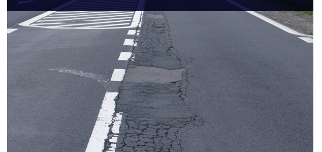
Fatigue cracking
