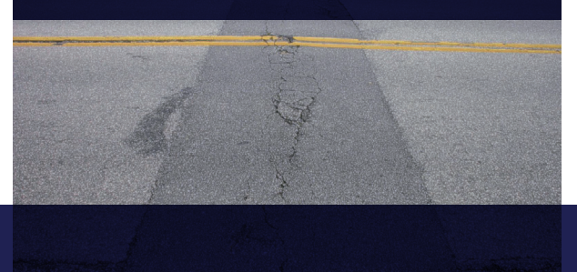
Reflective cracking
