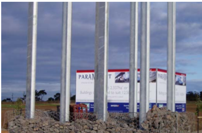
Main structure steel framework
