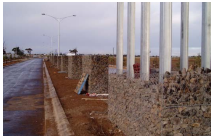
Gabion installation around the framework
