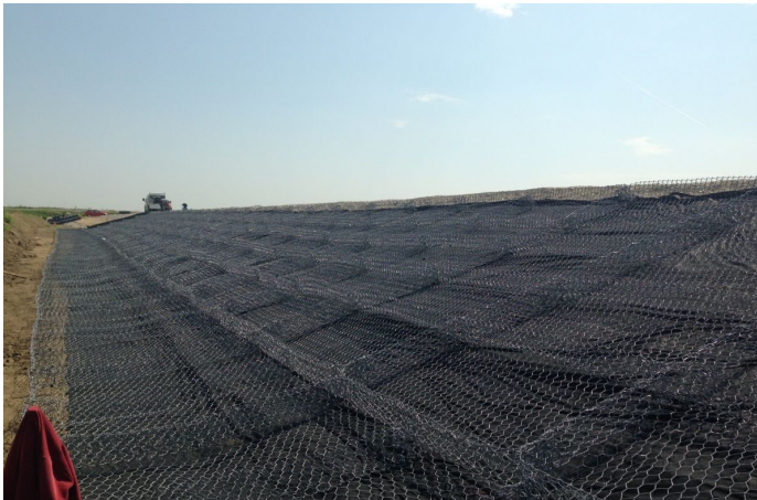
Installation phase: detail of the empty units
