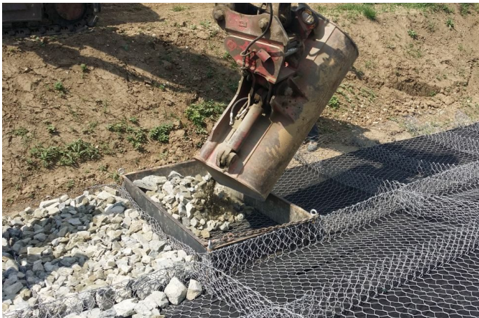
During the installation: stone-filling operation
