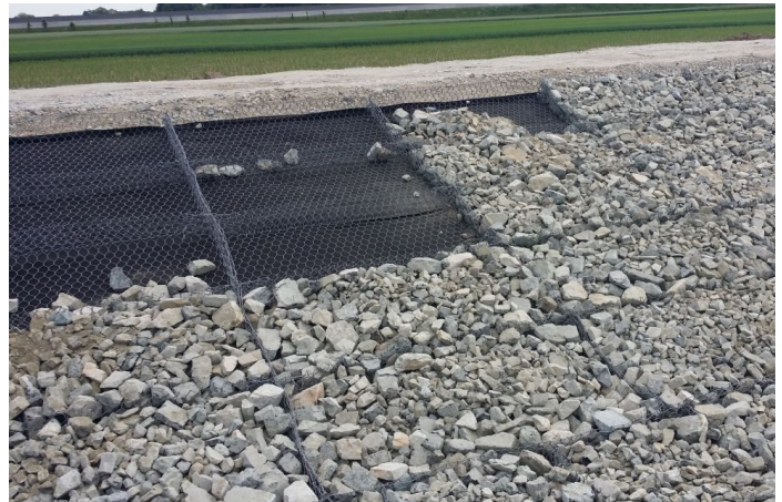
During the installation: stone-filling operation
