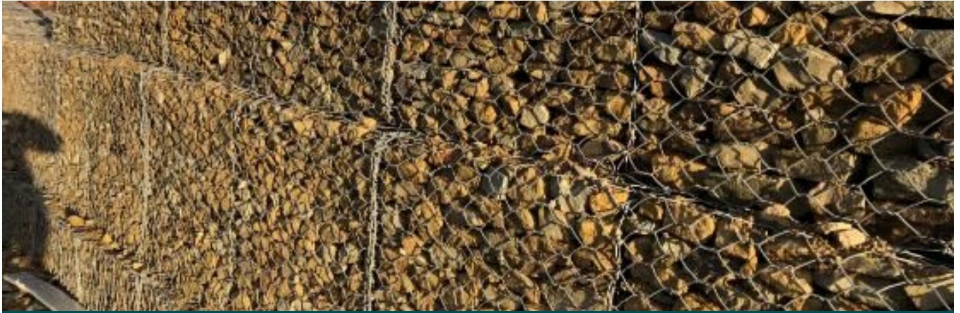
Gabion wall under construction
