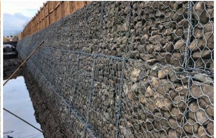
Finished Gabion wall
