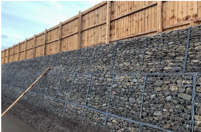
Finished gabion wall stretching along the line of properties
