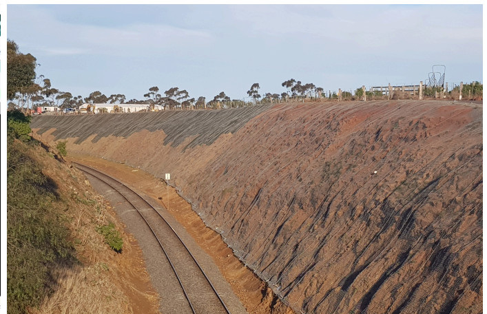
Completed Steelgrid rockfall mesh system
