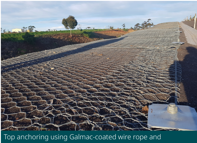
Installation of the Steelgrid® using rope access techniques
