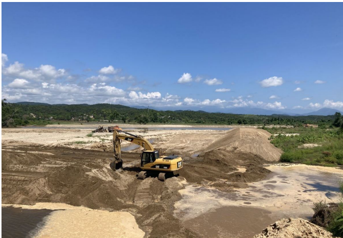
Starting of the works
