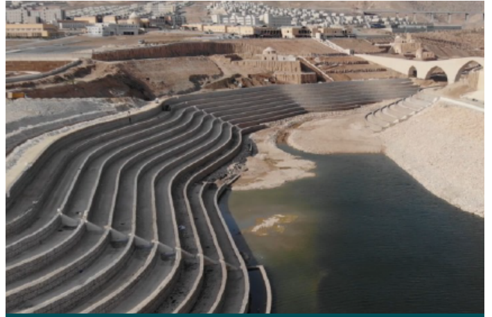
Terramesh System Walls
