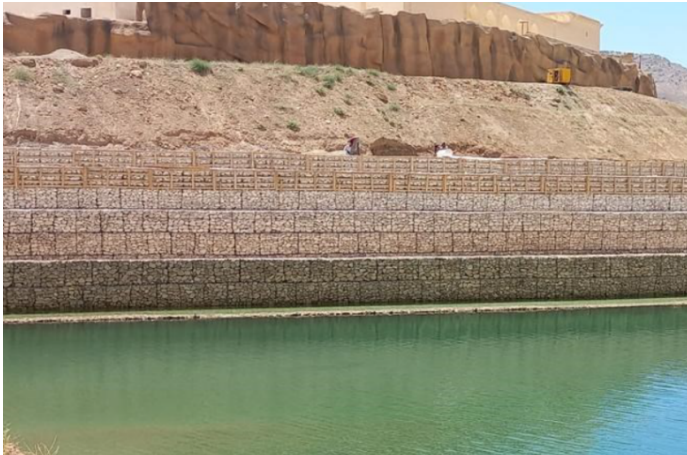
During Construction—After Rising of Water Level
