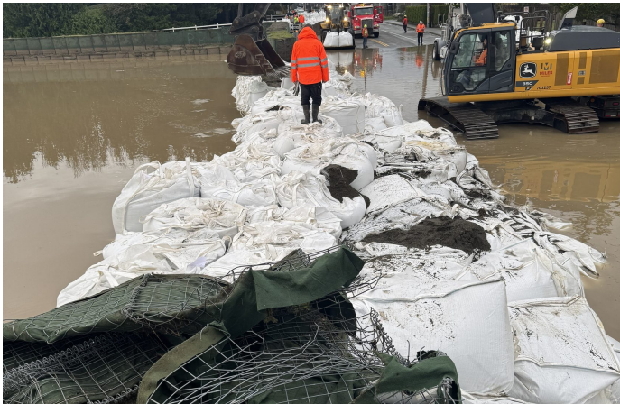
Before: Previous Breached Flood Barrier System
