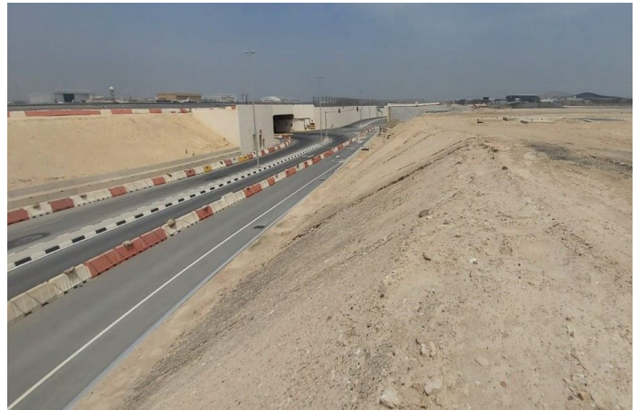
Slope before protection
