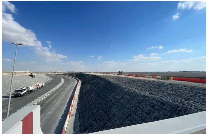
Completed Reno Mattress Lining
