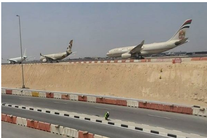
Slope before protection
