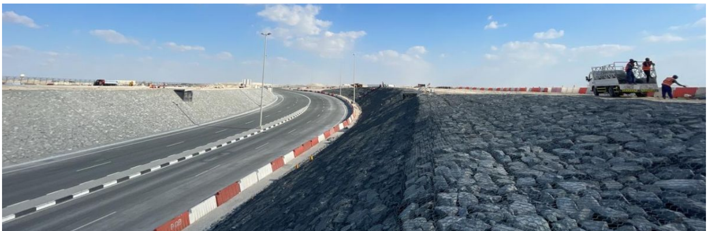
Steep slope protected with Reno Mattress
