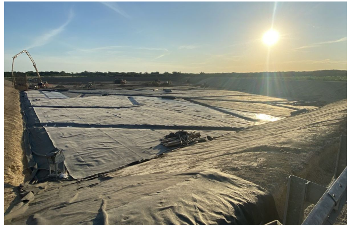
Starting of installation
