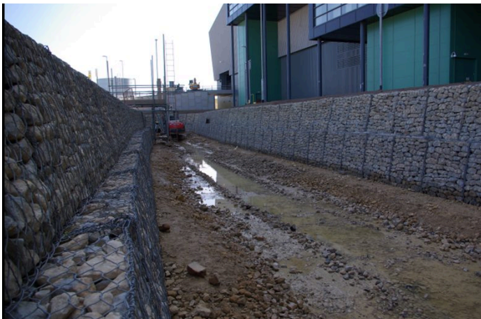
Installation of double twist gabions
