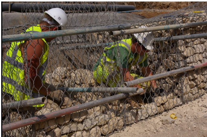
MacLine® and Gabion installation
