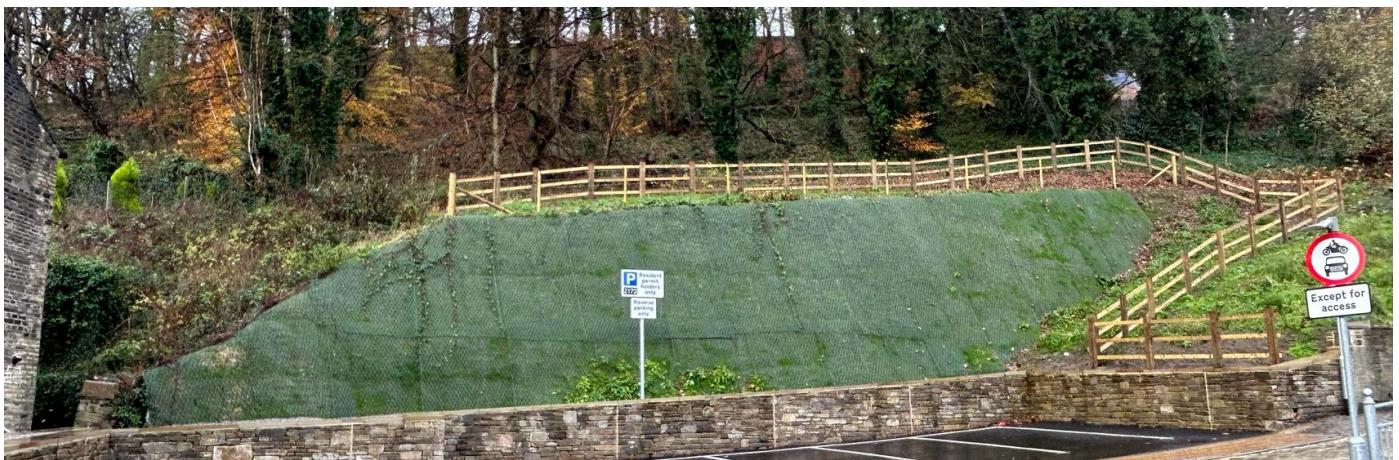
GeoMac system installed
