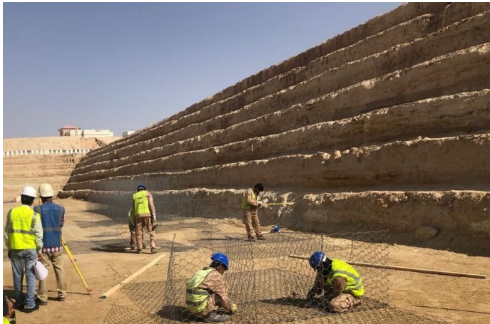
During construction : Excavation for pond construction
