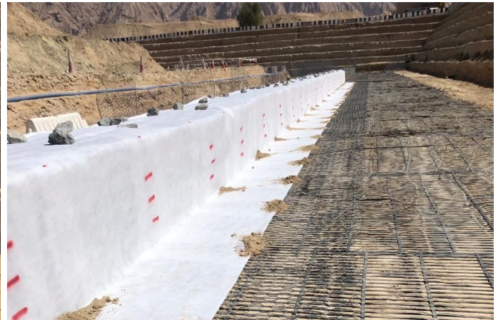
During construction : Geotextile &amp; Paragrid geogrid installed
