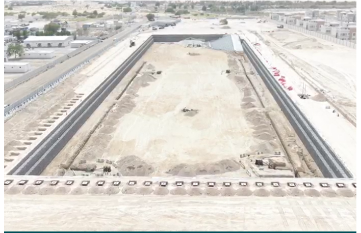
Completed pond : Before discontinuance of de-watering
