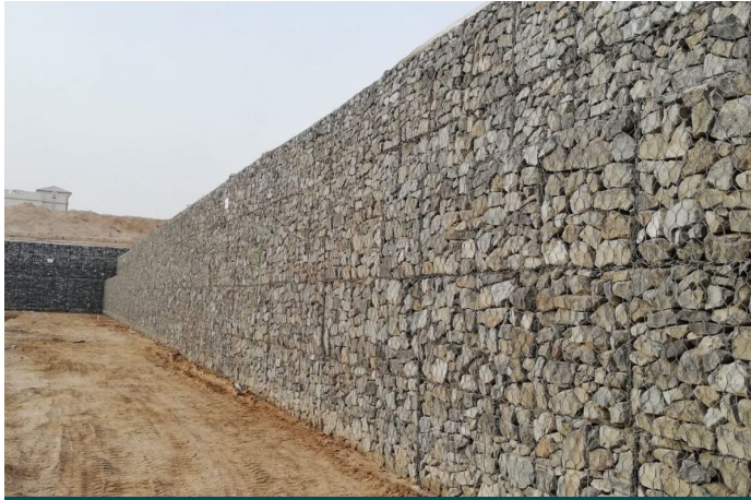
During construction : Terramesh wall in progress
