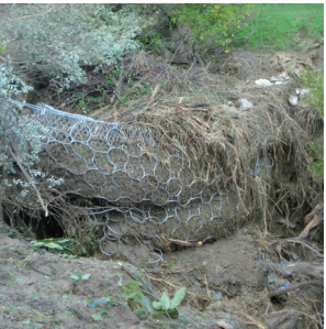
4 Debris Flow & Shallow Landslides
