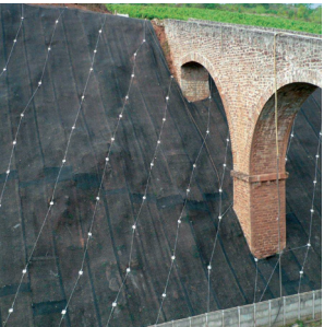
6 Soil Nailing and Surface Protection
