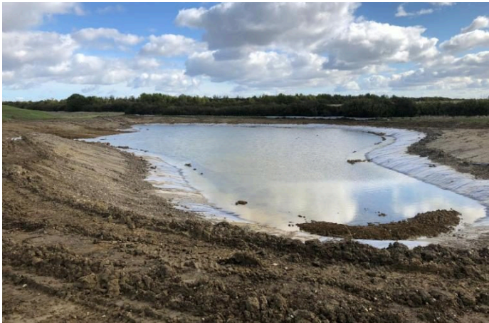
MacLine GCL lining in place post-construction
