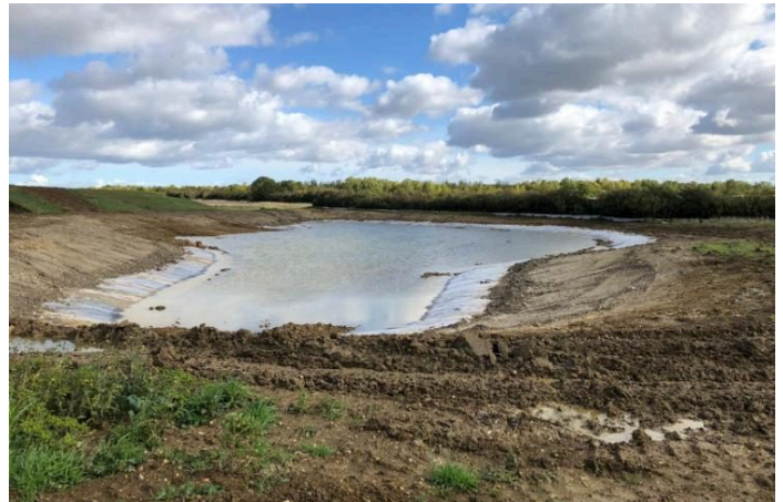
MacLine GCL lining in place post-construction
