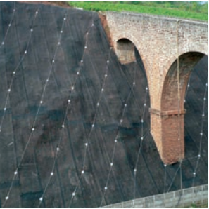
6 Soil Nailing and Surface Protection
