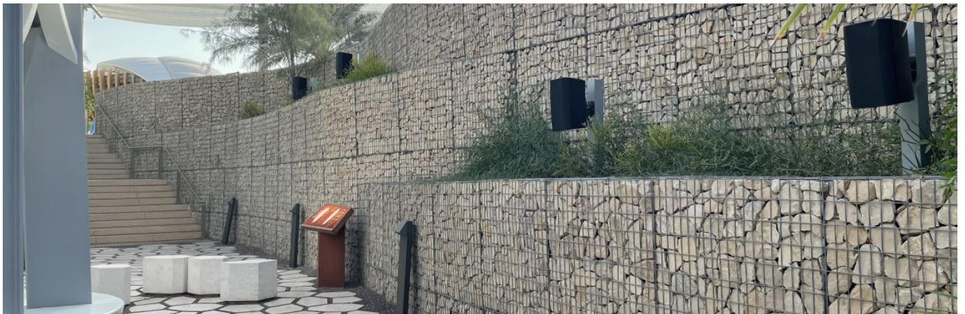
Completed weldmesh gabion wall in Dubai expo project
