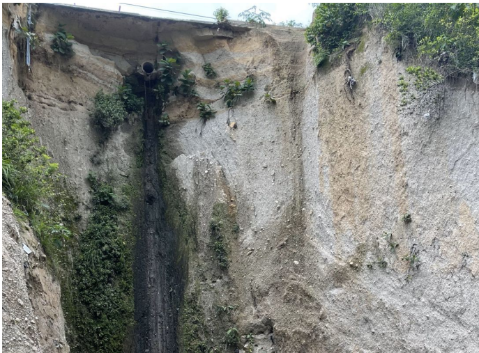
Before the construction
