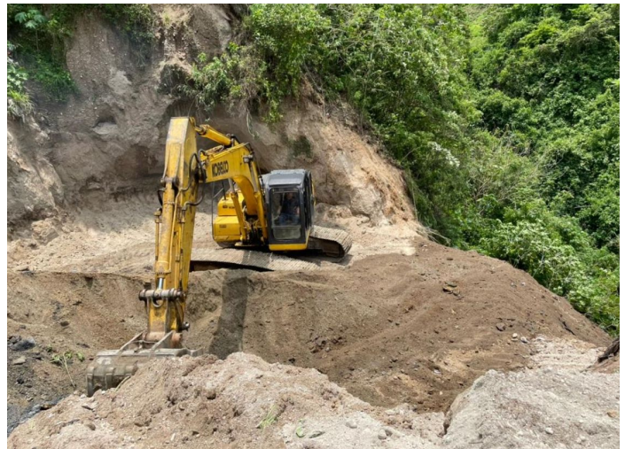
Starting of the works
