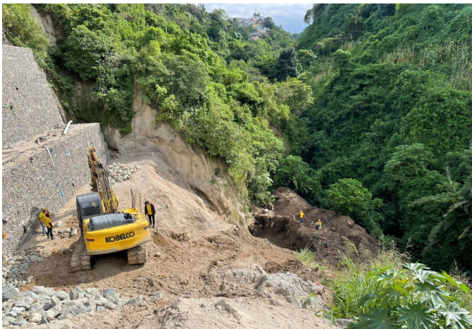
During the construction
