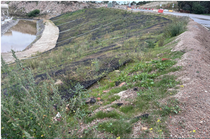
Vegetation Growth Two Months After Installation
