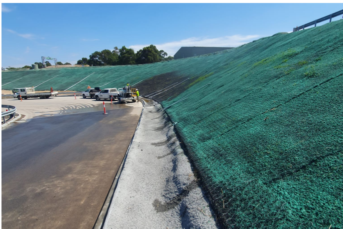
MacMat R Installation with Hydroseeding
