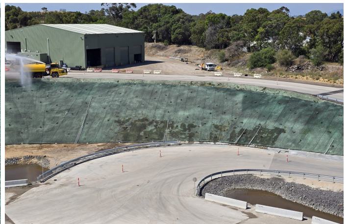
MacMat R Installation with Hydroseeding
