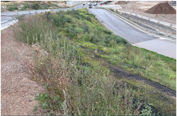
Vegetation Growth Two Months After Installation
