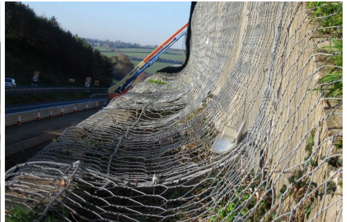
Steelgrid mesh anchored to the original slate formation.
