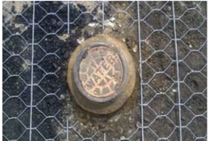
Roadmesh is cut to go around existing utilities
