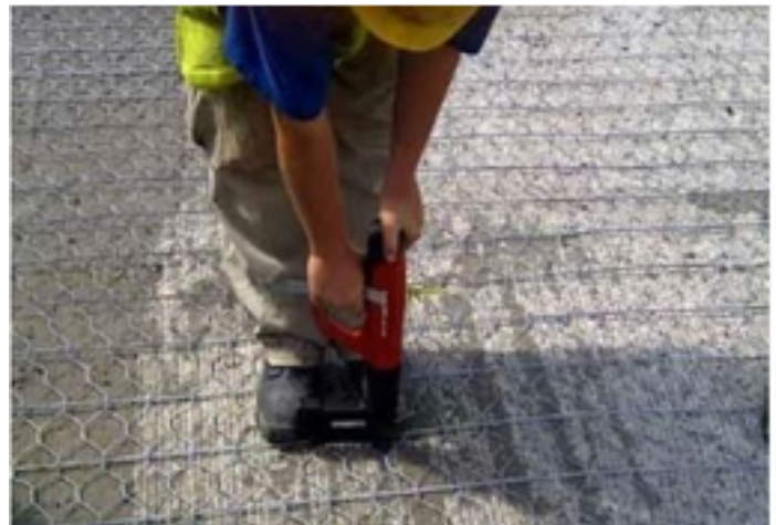
Roadmesh installation
