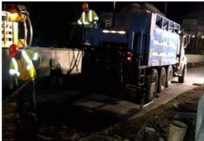
Slurry seal being placed on top of roadmesh
