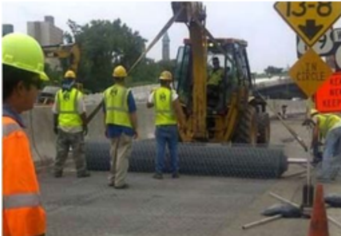
Rolling out the Roadmesh for placement
