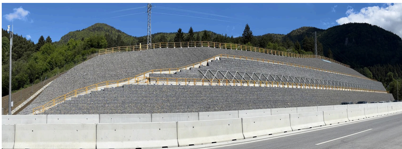
View of the finished work
