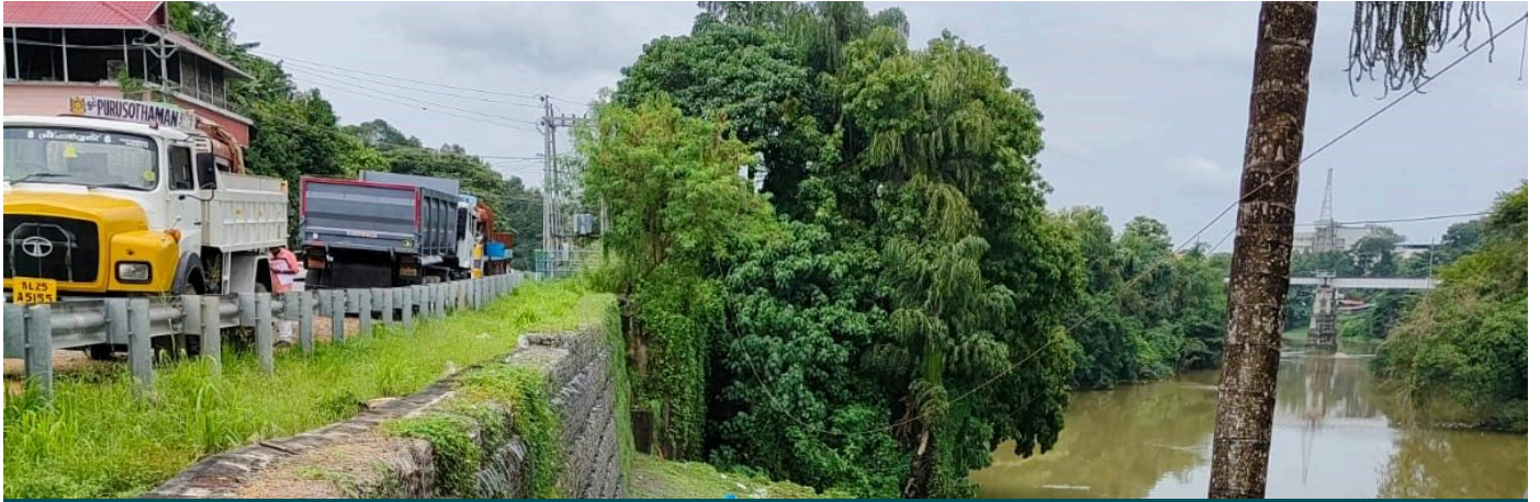
After Completion-Final Structure
