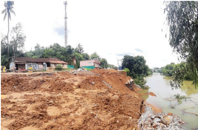
CONDITION BEFORE START OF WORK
