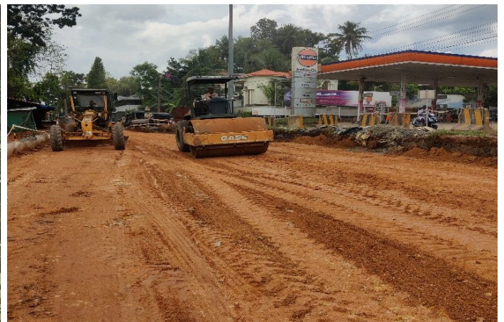
Compaction during construction
