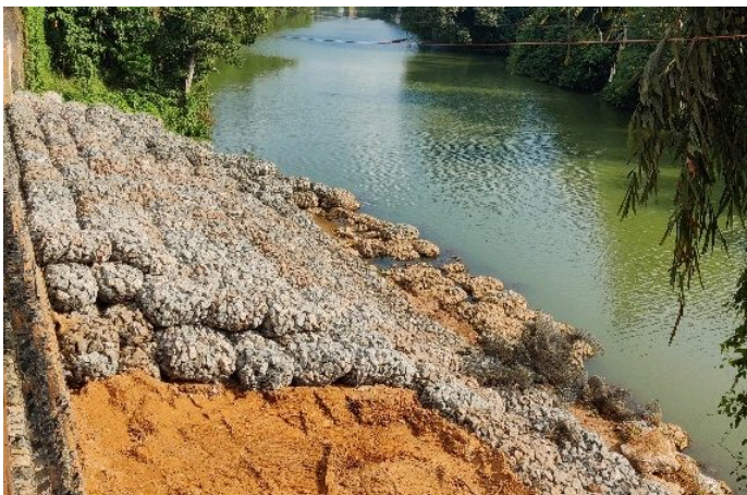
Placing of Sack Gabions as counter berm
