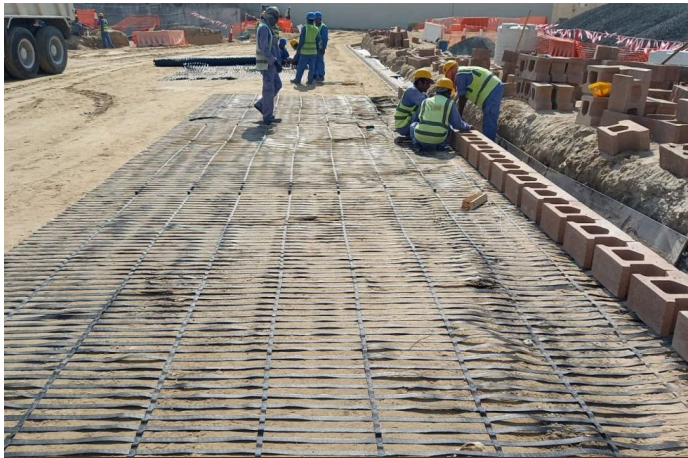
MacWall work in progress
