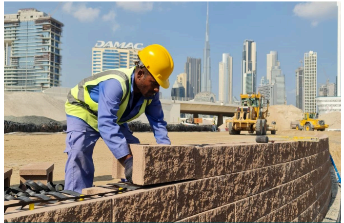
MacWall work in progress
