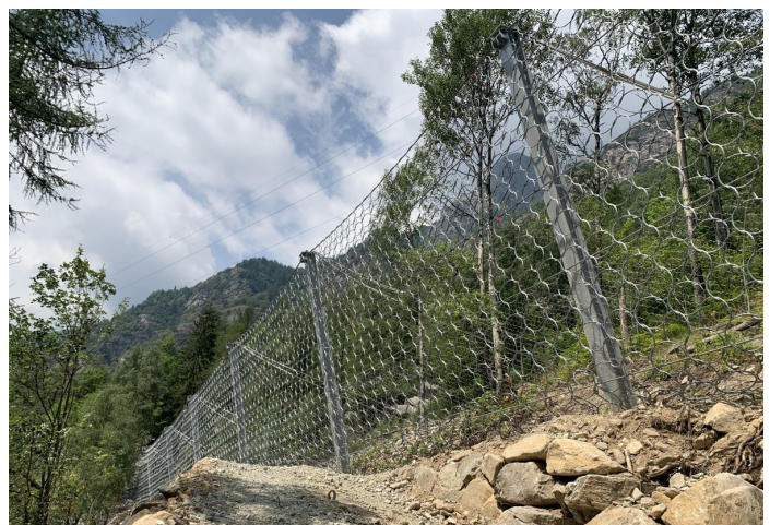
RB 9000 rockfall barriers installed – view from the valley
