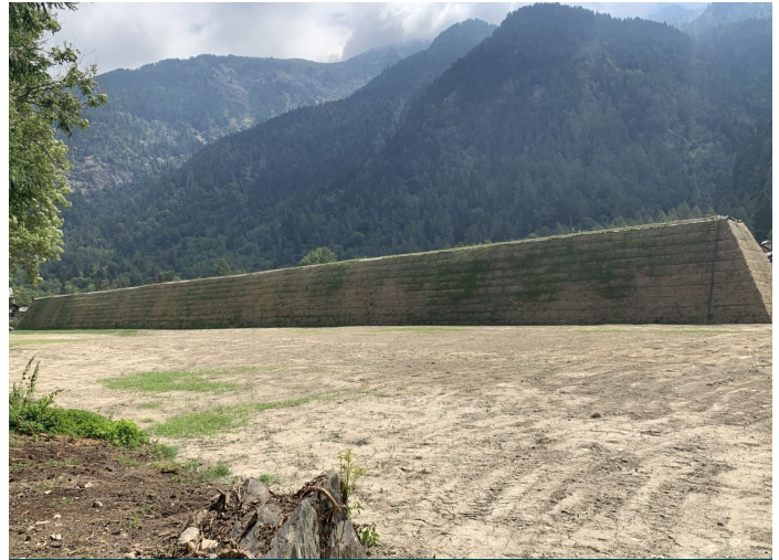
Rockfall barrier detected in Terramesh Verde, installed
