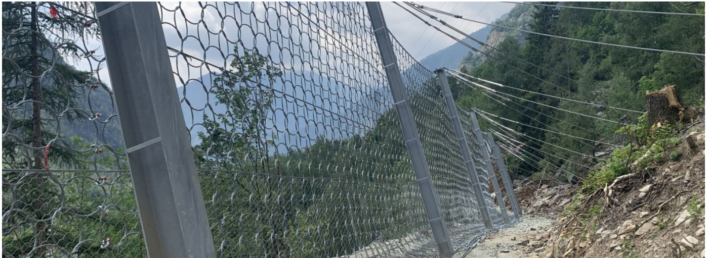
RB 9000 rockfall barriers installed – view from the uphill side
