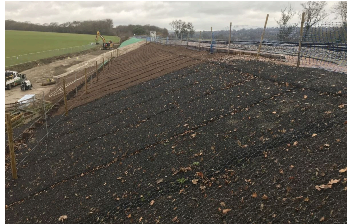
Topsoil dressed into the 3D matrix of the RenoMesh
