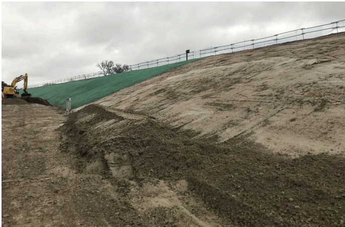
Anti Burrowing Mesh installed on the prepared embankment
