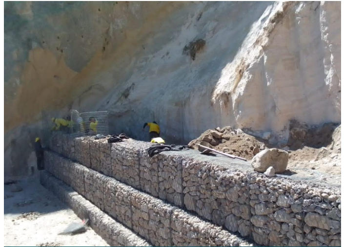
Starting of construction
