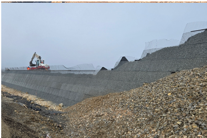
Mineral Terramesh® Construction Underway
