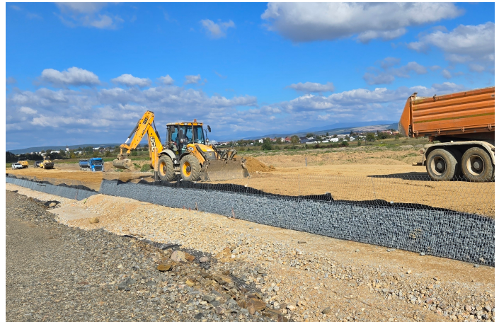
Installation of the first row of the Mineral Terramesh® system
