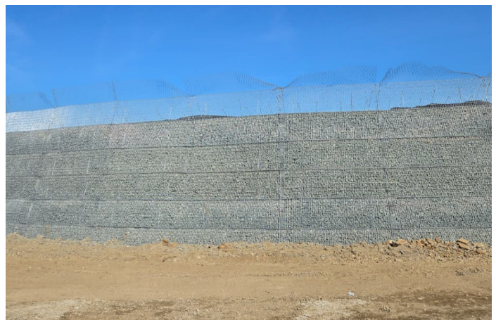
Mineral Terramesh® Construction in an Arch
