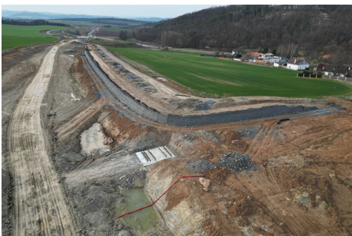
Top view of the Mineral Terramesh® structure
