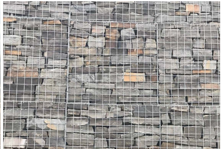
Maccaferri Construction hand placed the selected slate stone
