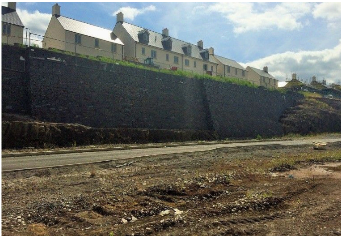
Welded gabion installed in Coed Darcy
