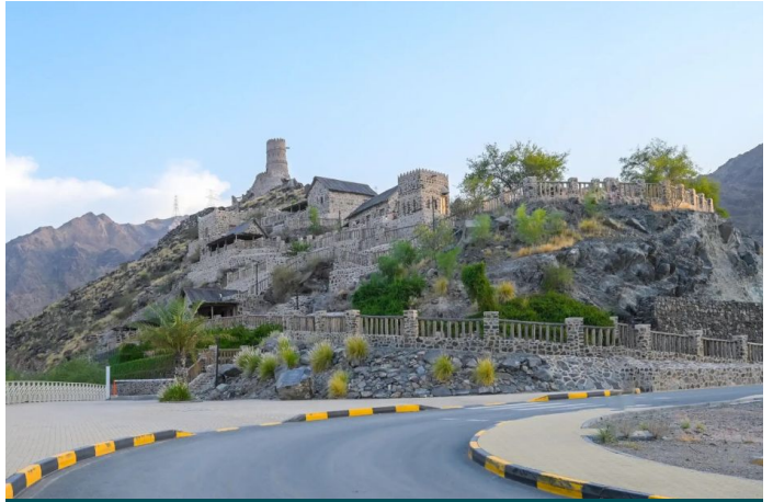
Completed Terramesh wall seamlessly integrated with the
