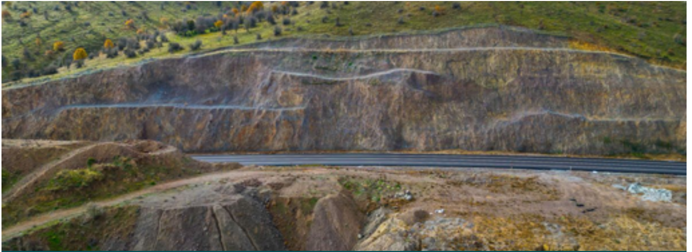
RINGNET INSTALLATION ON SLOPES
