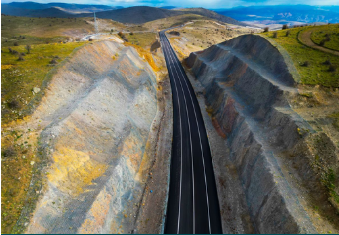
RINGNET INSTALLATION ON SLOPES
