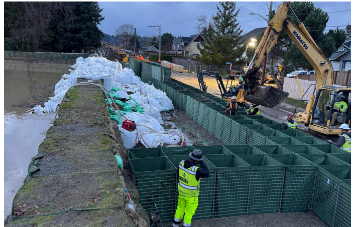
During: Emergency Breach Repair
