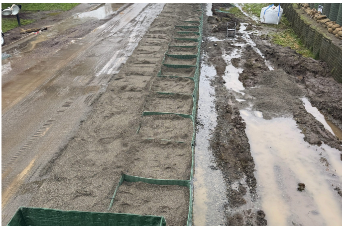
During: Emergency Breach Repair Protecting Pacific Park
