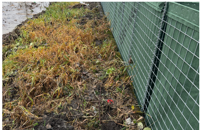
After: White River Flood Protection Barriers
