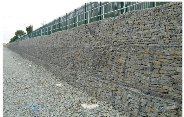
Start of construction
