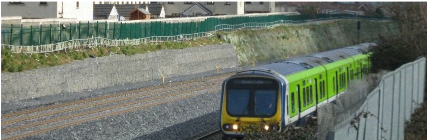
MacMat® R and soil nails after hydroseeding
