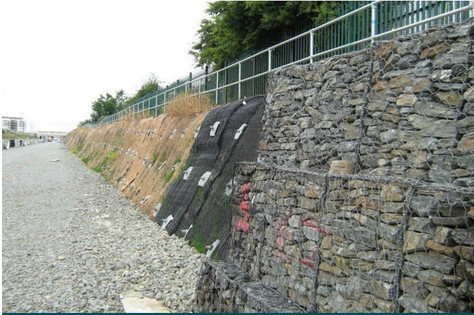
Installation of Gabion retaining wall
