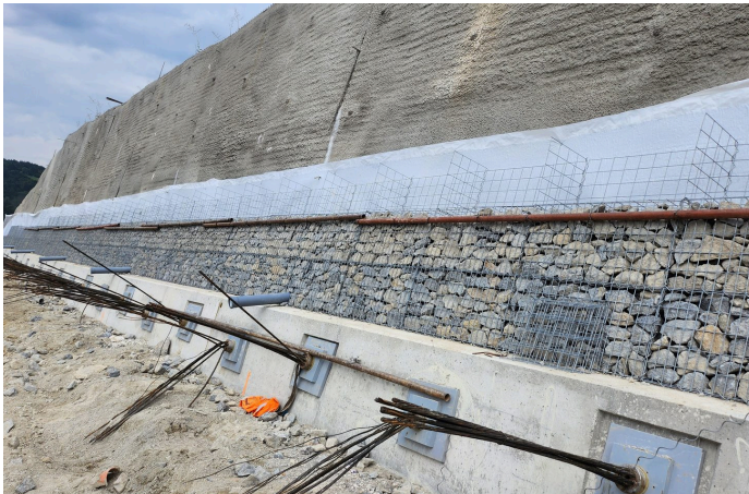
Installation of gabion facing
