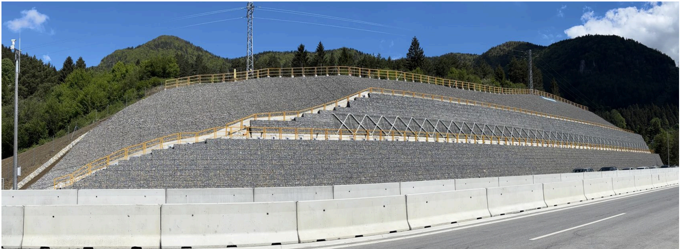
View of the finished work
