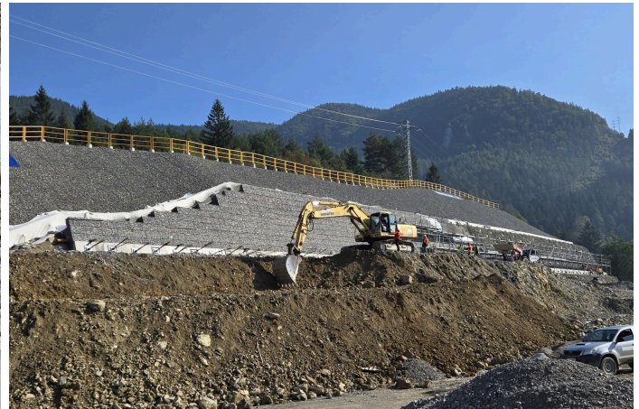
Installation of gabion facing
