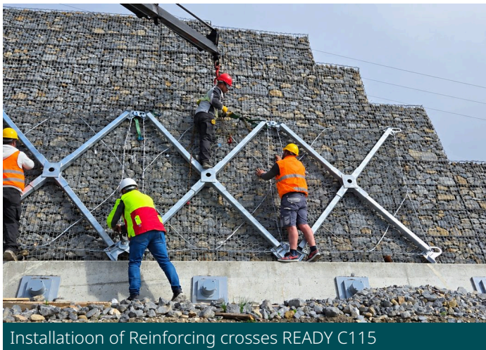
Installation of Reinforcing crosses READY C115
