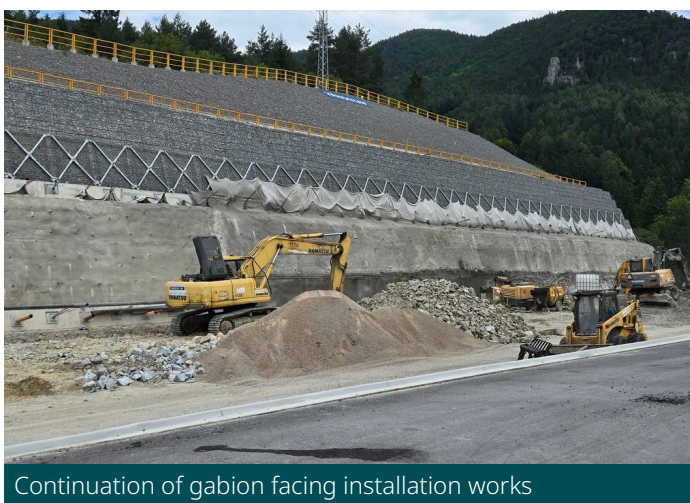
Continuation of gabion facing installation works
