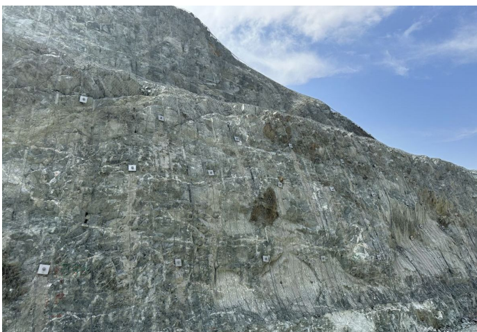
Completed: Secured drapery with Steelgrid HR mesh
