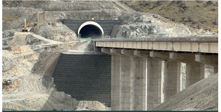
Completed: Terramesh MSE wall at bridge and tunnel portal
