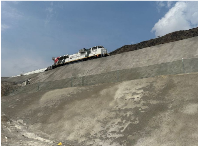
Completed: Shotcrete covered slope reinforced with Paragrid
