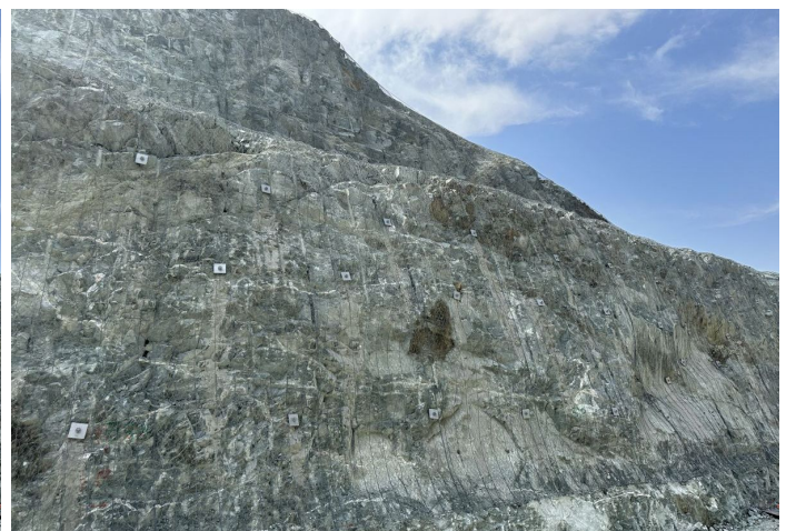
Completed: Simple drapery with Steelgrid HR mesh.
