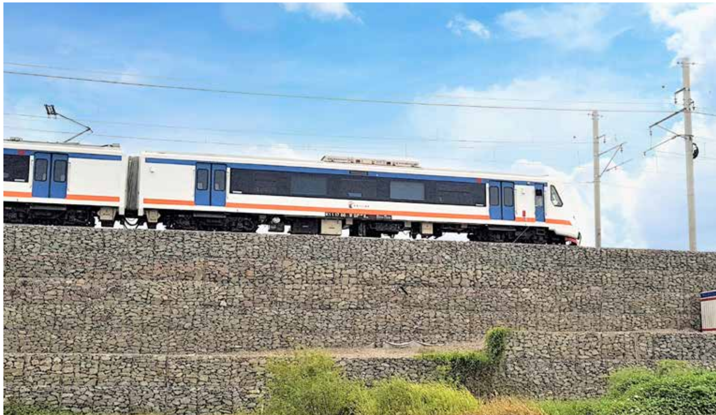
Paramesh - Bandara Soekarno-Hatta Railink, Jakarta
