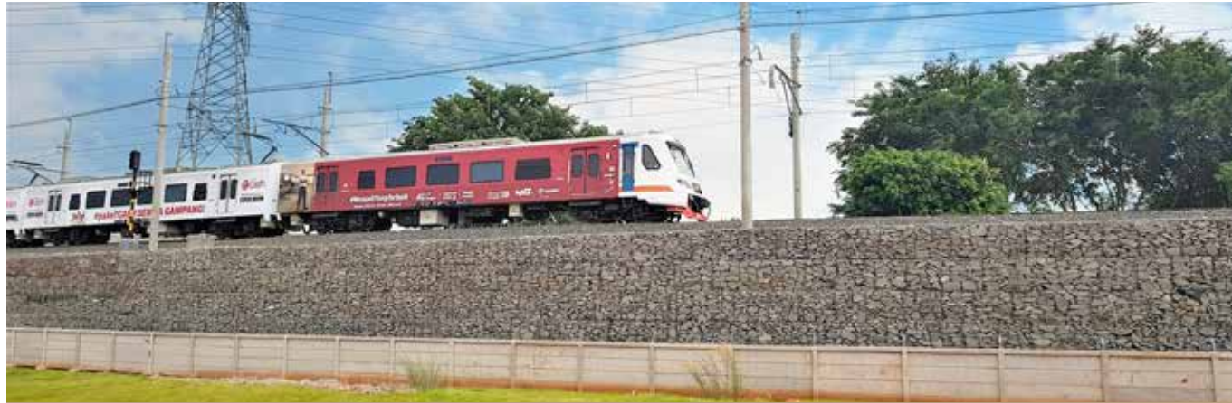
Paramesh - Bandara Soekarno-Hatta Railink, Jakarta
