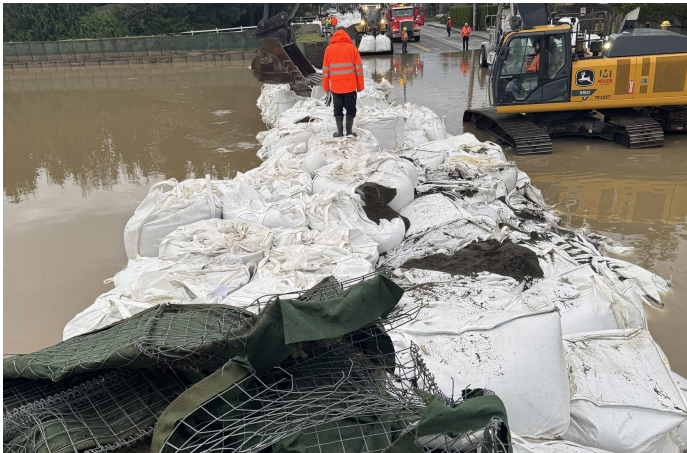
Before: Previous Breached Flood Barrier System
