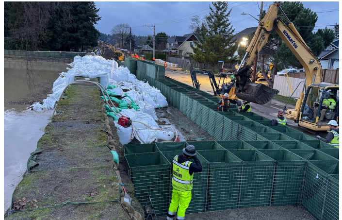
During: Emergency Breach Repair
