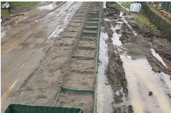
During: Emergency Breach Repair Protecting Pacific Park
