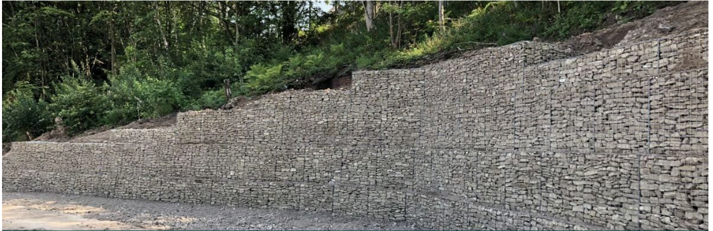
Different stone fill types used to create stripes of darker stone
