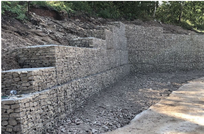
Welded gabion wall nearing completion
