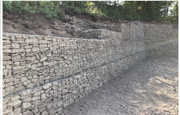
Corner detail of welded gabion wall
