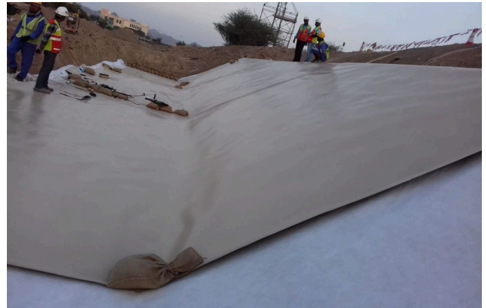
During construction: Beige colour HDPE geomembrane
