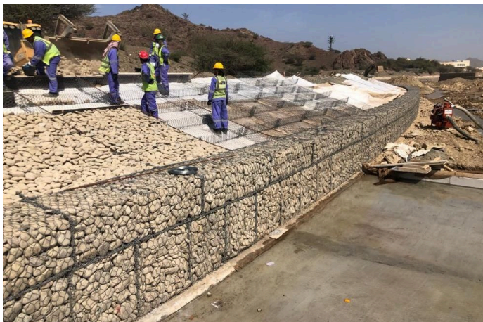
During construction: Polimac coated gabion mattress
