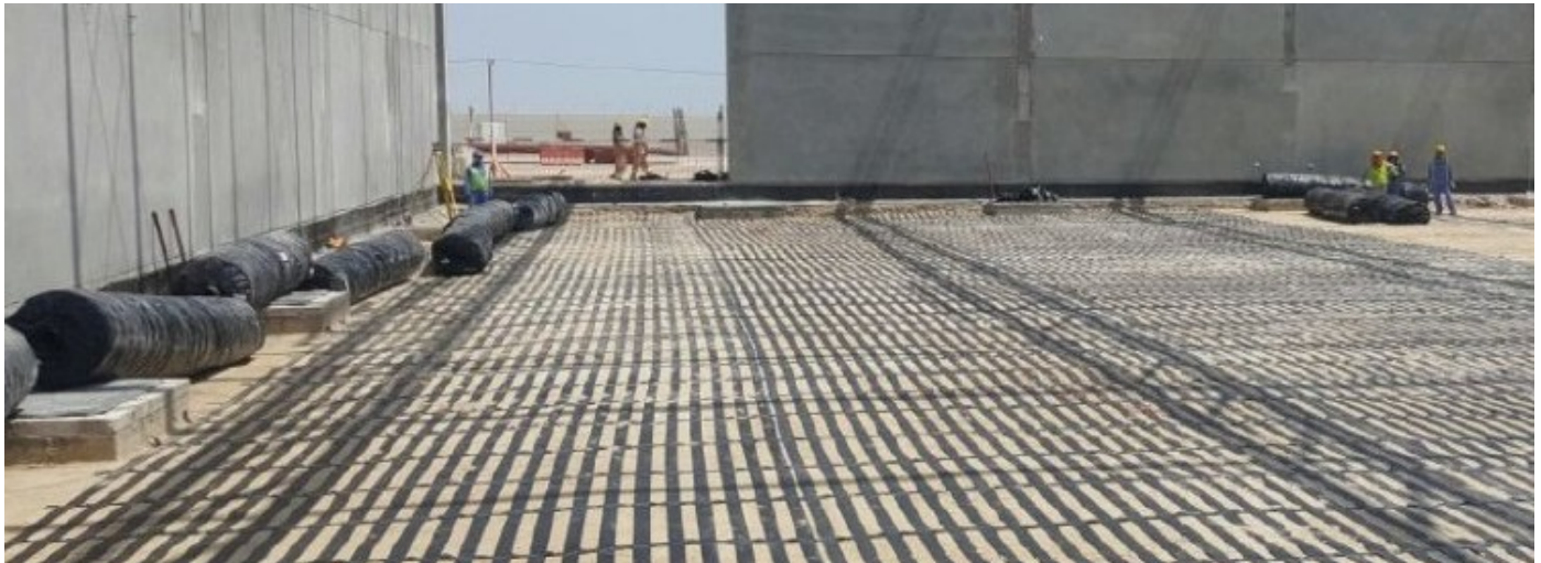
SPENT POT LINING (SPL) STORAGE BUILDING - EMAL
