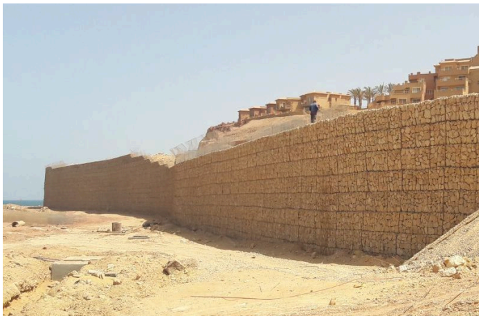
During construction: Paramesh MSE wall installation in
