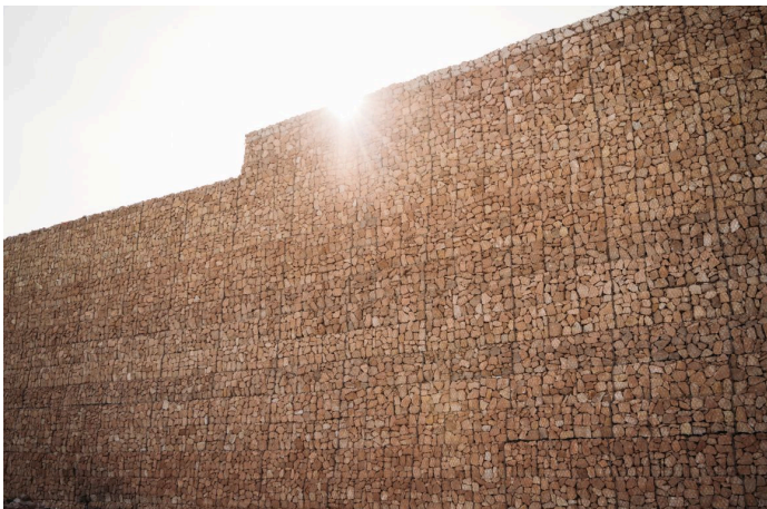
Completed: close view of Paramesh MSE wall
