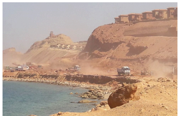
During construction: initial site activities
