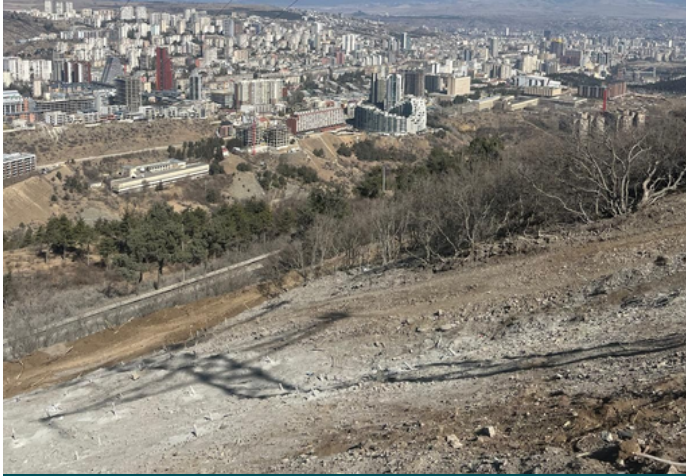
Pre-Installation Condition of the Slope
