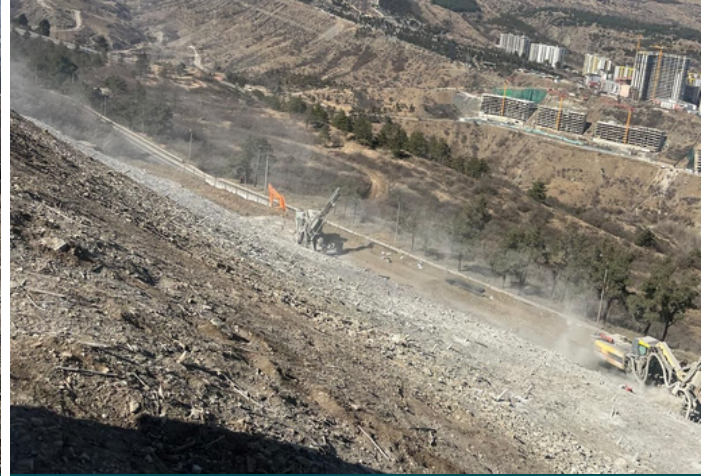
Pre-Installation Condition of the Slope
