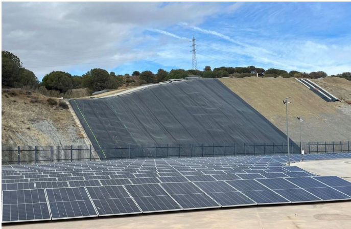
Installation of the double-twisted mesh
