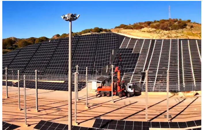
Solar panel installation process on the slope
