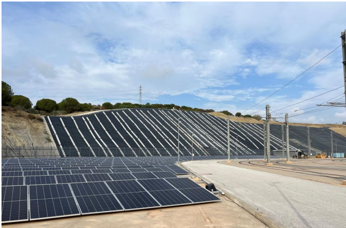
Complete installation of the mesh
