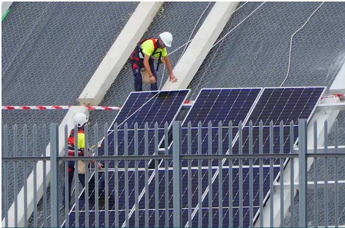
Solar panel installation process on the slope
