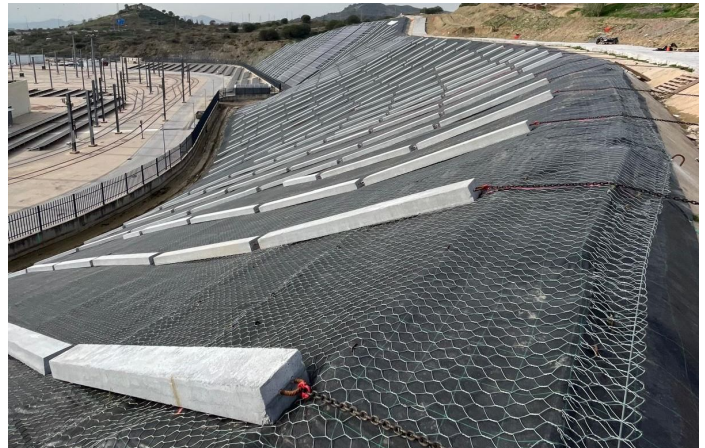
View from the crest during the construction process
