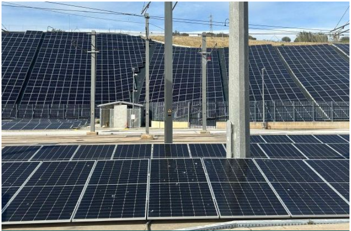
Completion of the third phase of the photovoltaic solar plant
