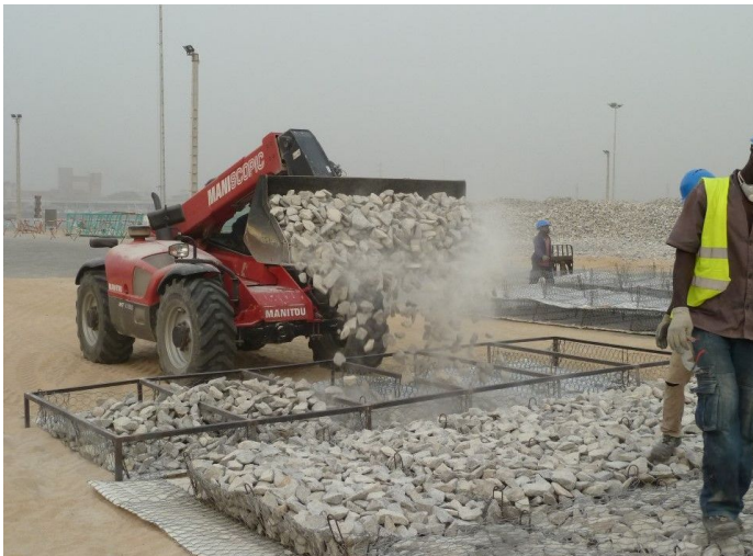
Filling of the Reno Mattresses
