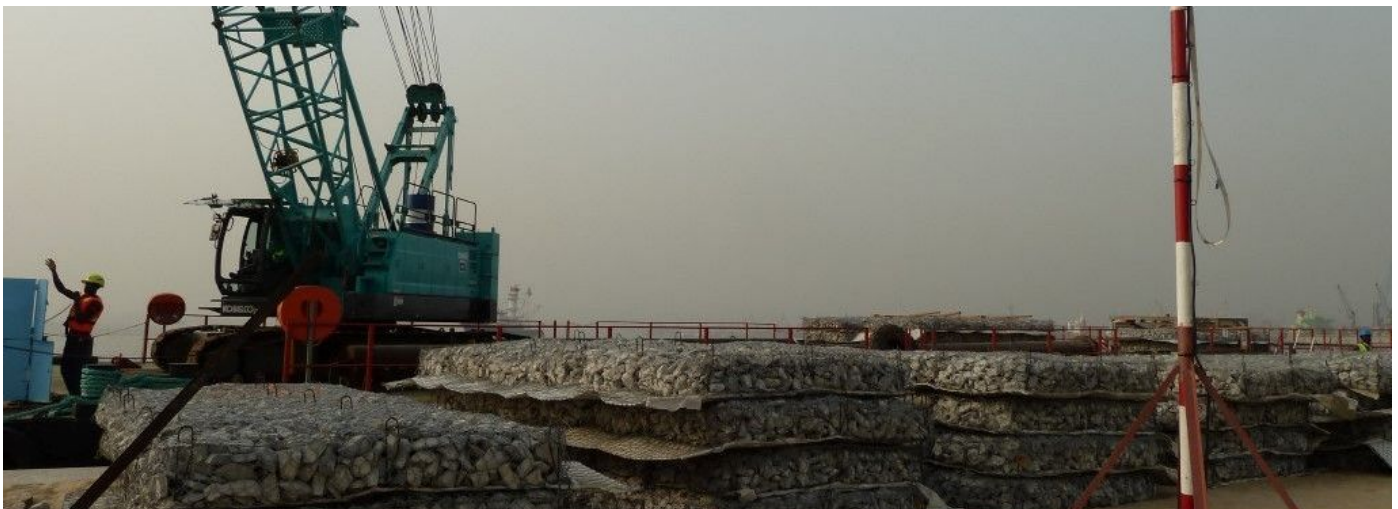
Placement of the Reno Mattresses
