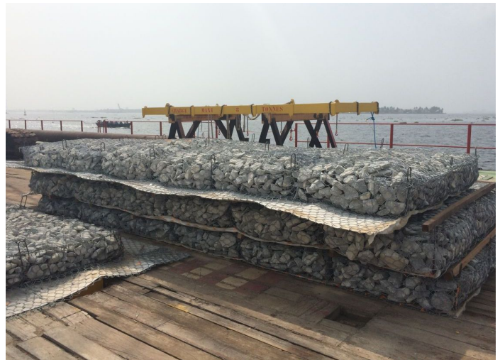
Placement of the Reno Mattresses
