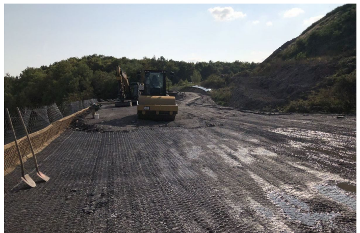
Construction phase: laying of Terramesh units
