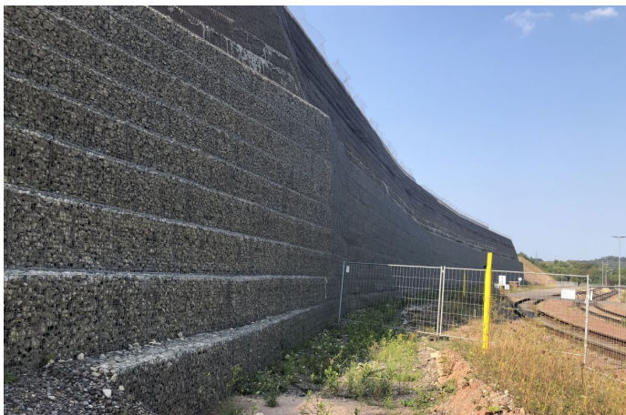
End of the construction: side view
