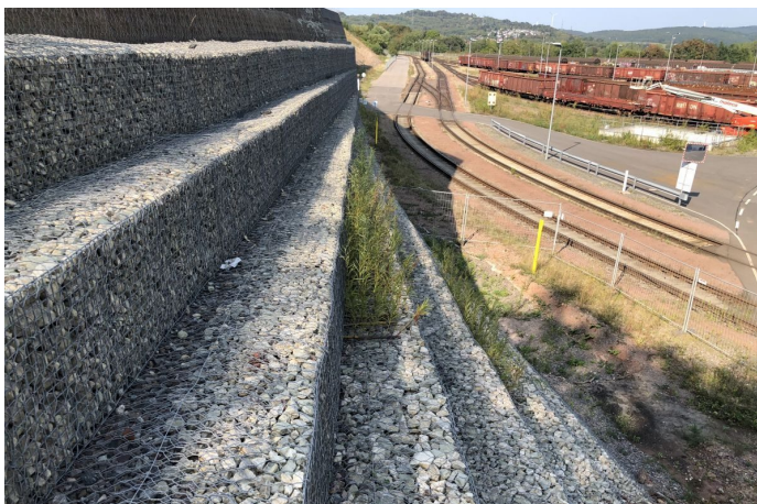
Construction phase: side view
