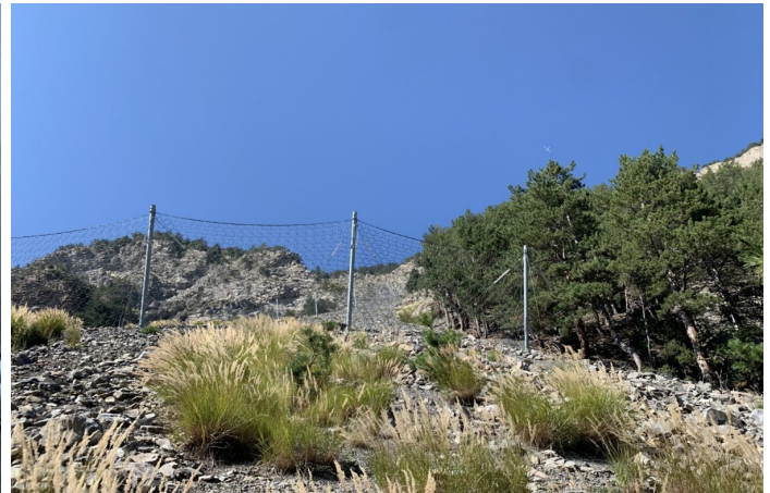
Dynamic rockfall barriers installed
