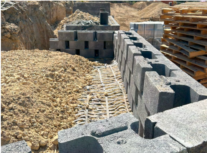
ParaGrid geogrid reinforcement used for MacWall
