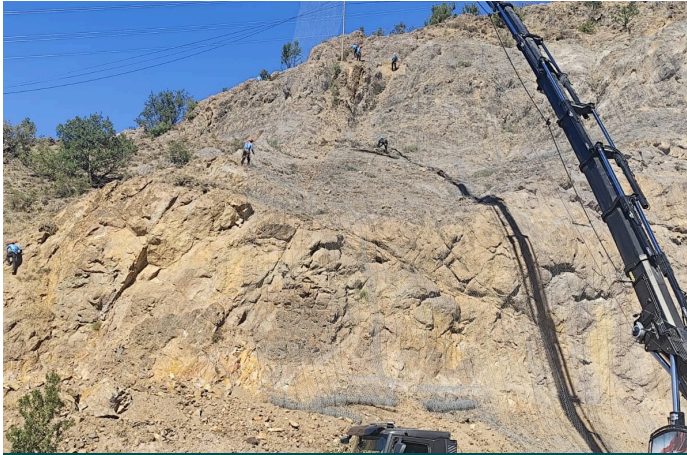
During the construction
