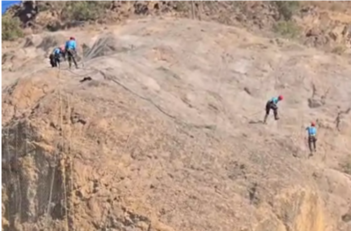
During construction – installation of surface anchors
