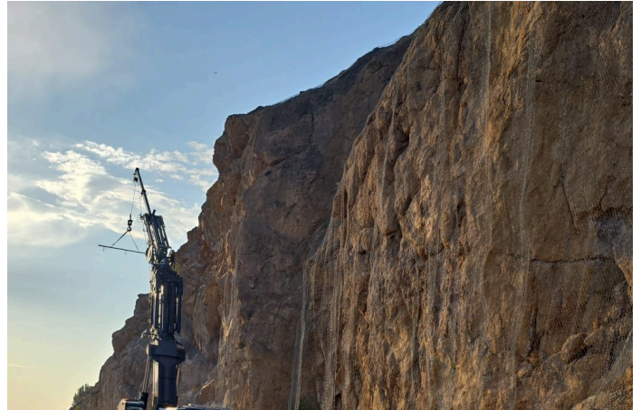
After the construction
